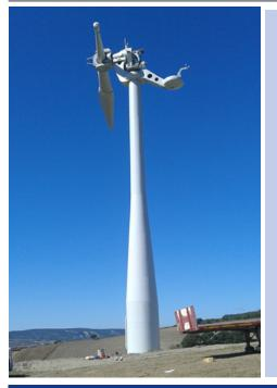
Although the wind turbine can be installed on a conventional tubular tower, its special features allow it to be mounted on a lattice tower. This is mainly due to the fact that the motor torque of the turbine is absorbed by mechanical elements that prevent the bending moment from being transmitted to the tower. Therefore, the tower only bears wind stress and stress derived from the weight of the nacelle.
